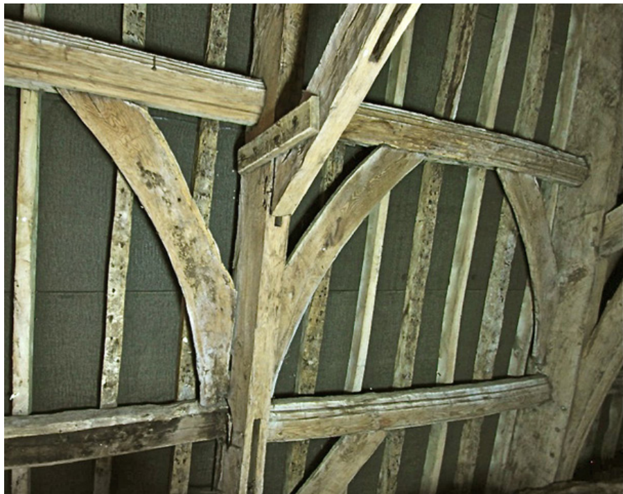
Fig. 7b Milborne Port, 14-17 High Street, Detail of the purlins and wind braces, also empty arch-brace mortices
