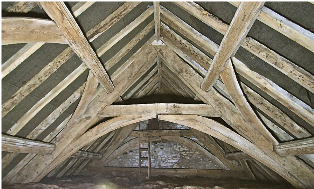
Fig. 7a Milborne Port, 14-17 High Street, The west end of the high quality arch- and wind-braced roof
