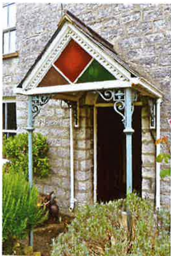
Fig. 11 Kingsbury Episcopi, The Retreat, porch canopy on cast iron supports
