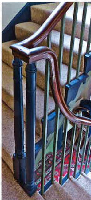
Fig. 8 Kingsbury Episcopi, Manor House. Ramped handrail and decorative brackets to treads
