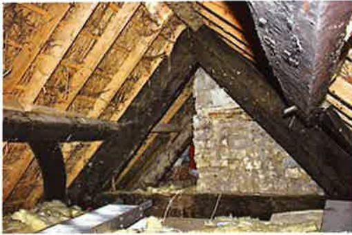
Fig. 5 Kingsbury Episcopi, West Lambrook, Tanyard House. Smoke-blackened truss, purlins and windbrace
