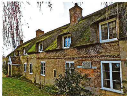
Fig. 12 Stocklinch, Ilford Bridges, front elevation displaying decorative brickwork
