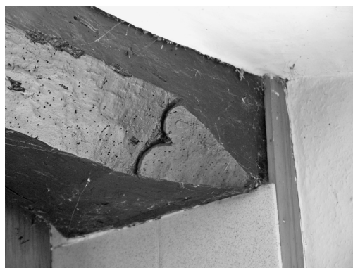
Fig. 2 High Ham, Henley Farm, detail of beam stop
