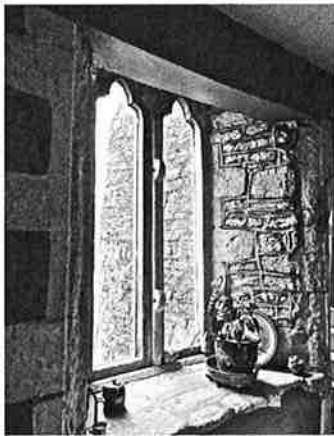
Fig. 5 14th-century window: Emborough, Manor Farm (photo John Rickard)
