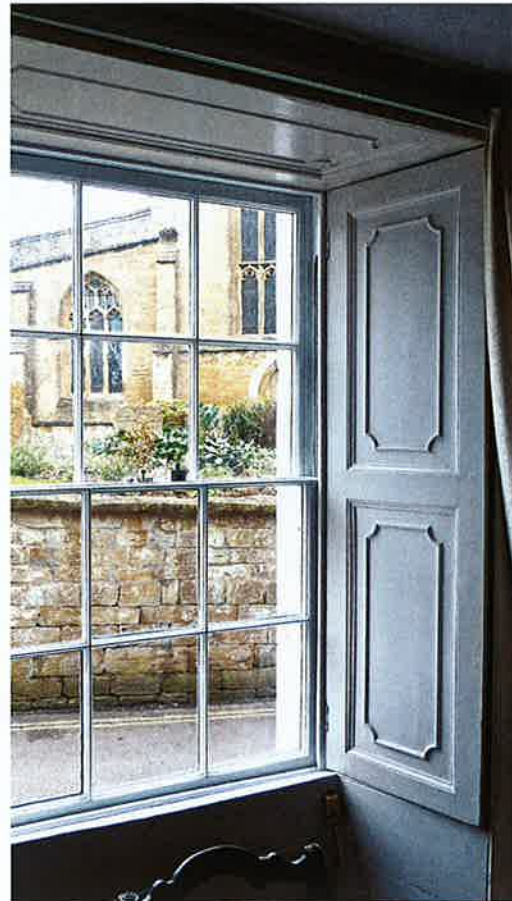
Fig. 22 South Petherton, 1 West St, shutters with applied beading
