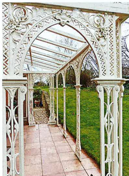
Fig. 20 South Petherton, Coles Lane, 1877 Coalbrookdale iron verandah
