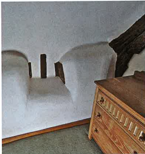
Fig. 5 Dowlish Wake, Mount Cottage: supposed wind-eye
