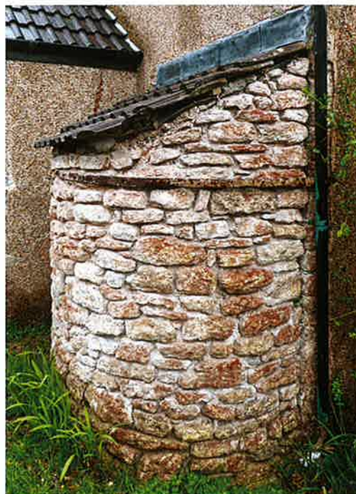
Fig. 14 Rodney Stoke, Hollybrook Farmhouse, housing for an added oven
