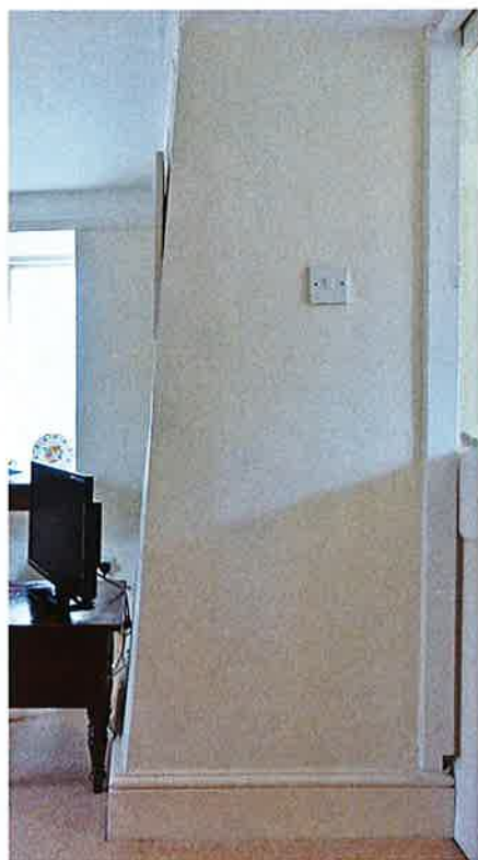
Fig. 18 Rodney Stoke, Stoke St, The Anchorage, wall batter
