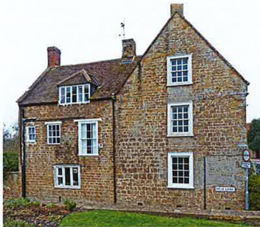
Fig. 21 South Petherton, 1 West St, east gable with false chimney
