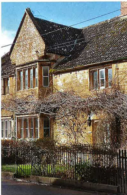
Fig. 8 Martock, 9 and 11 Hurst, the two-storey bay with corbelled gable
