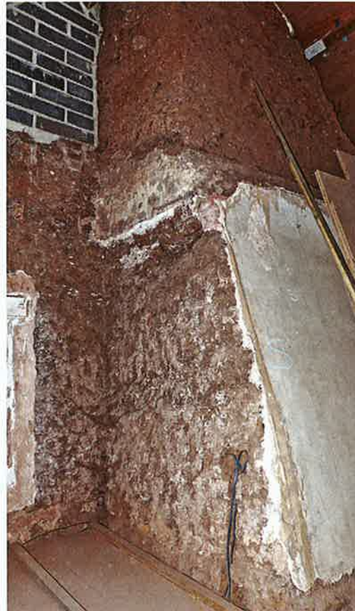
Fig. 1 Chilton Trinity, Braddocks Cottage. The enormous cob chimney as seen on the first floor
