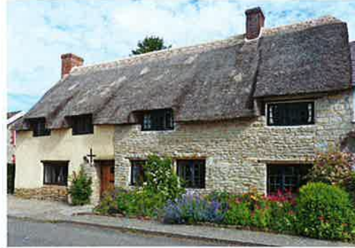
Fig. 12 Rimpton, Brambly Cottage
