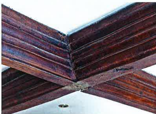
Fig. 9 Martock, 9 and 11 Hurst, moulded beams in framed ceiling
