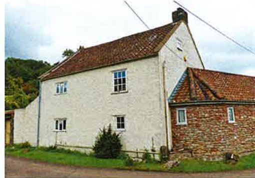
Fig. 17 Rodney Stoke, Scadden's Lane, Scadden's House, rear elevation
