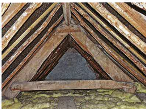
Fig. 13 Rodney Stoke, Holly Farm. Pole rafters of un-squared timber
